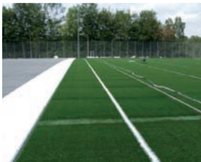
7 | Installation of artificial turf layers with integrated midline
