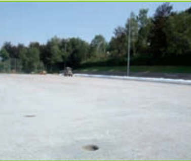
1 | Sub base with gravel surface
