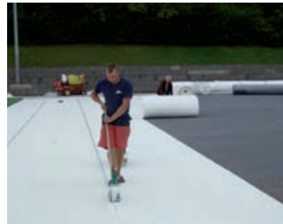
5 | Welding of roll joints with adhesive tape
