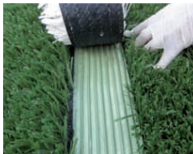
12 | Gluing of lines
