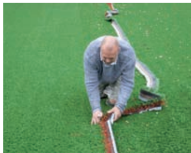
8 | Cutting of artificial turf edges
