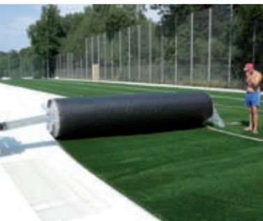
6 | Installation of artificial turf layers on ProGame shock pads
